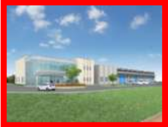
Hydrogen Energy Test & Research Center (HyTReC)
